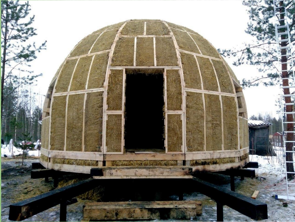
Straw dome 6,5 meters of inner diameter(individual project) near Saint Petersburg, Russia 2016
